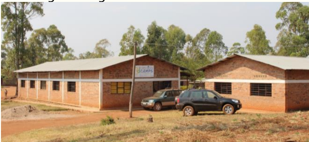
Just 2 of the 6 roofs that need painting/replacing and guttering.
